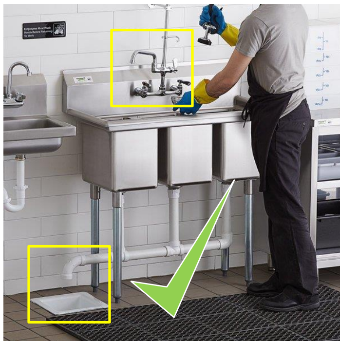
Required Two Airgap Design Into Floor Sink.
